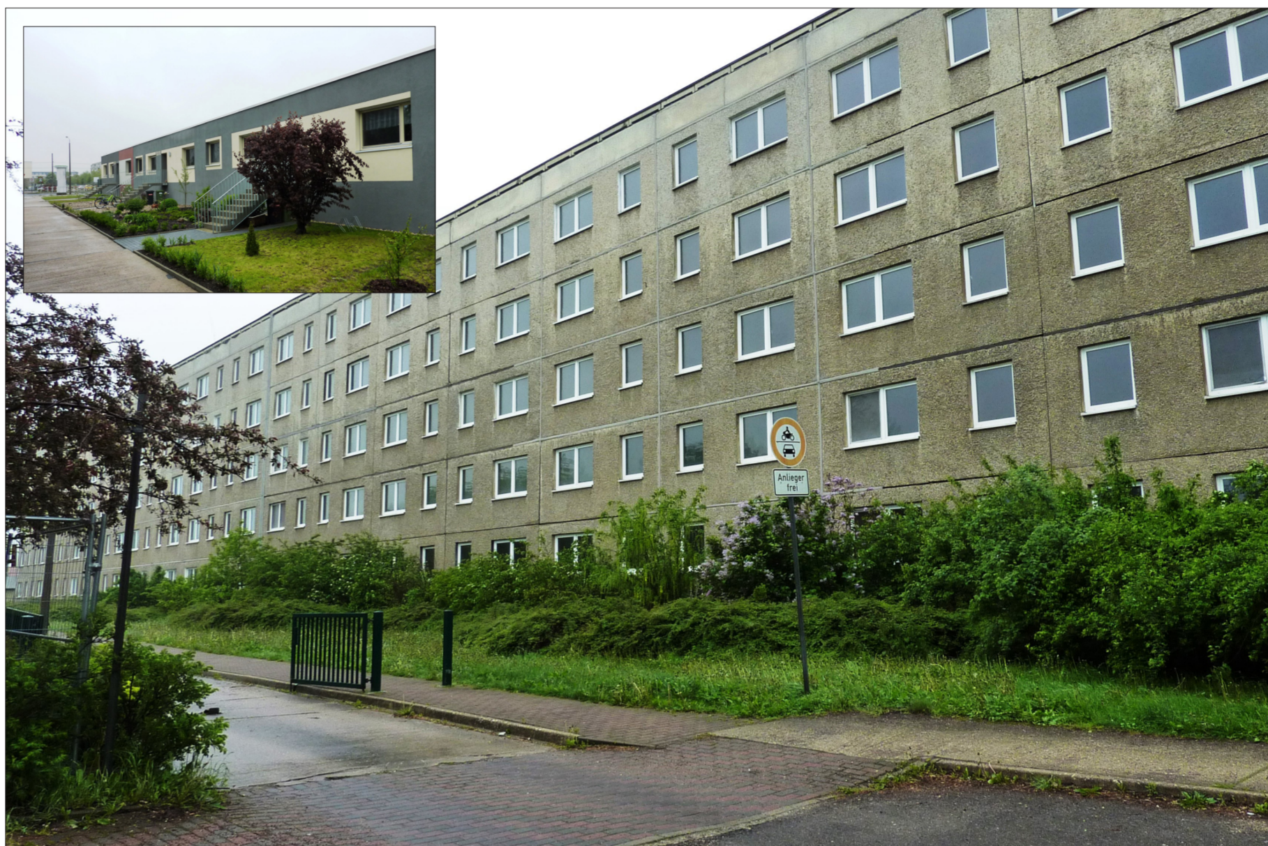
Transforming a Soviet-style block of flats into terraced single-story houses: Dessau, Saxony-Anhalt, Germany, May 2010.
