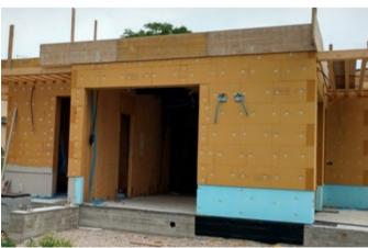
05-06 | Demonstrator building, Benevento. Construction phases: assembly of X-Lam panels (Cross Laminated Timber) and stratification of the external walls. The choice of the Fibertherm Flex 180 panel contributes to ensure a good thermal inertia thanks to its mass, making it suitable for the reference climate context
